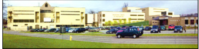
Waukesha County Correctional Facility
